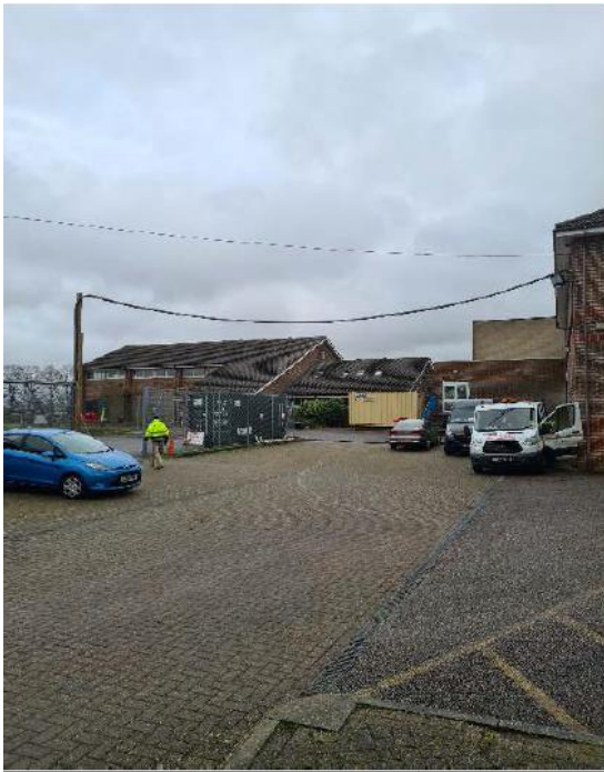
Creation of the new Sports Hall in progress
